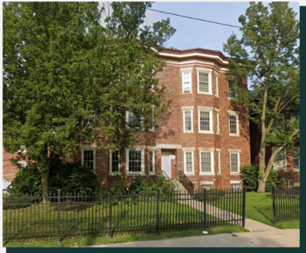
Algonquin Apartments 12 Units Warren - Conner
