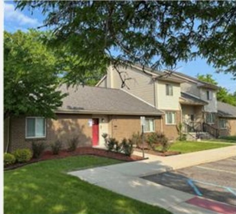
Brewster Homes 250 Units | Brush Park
