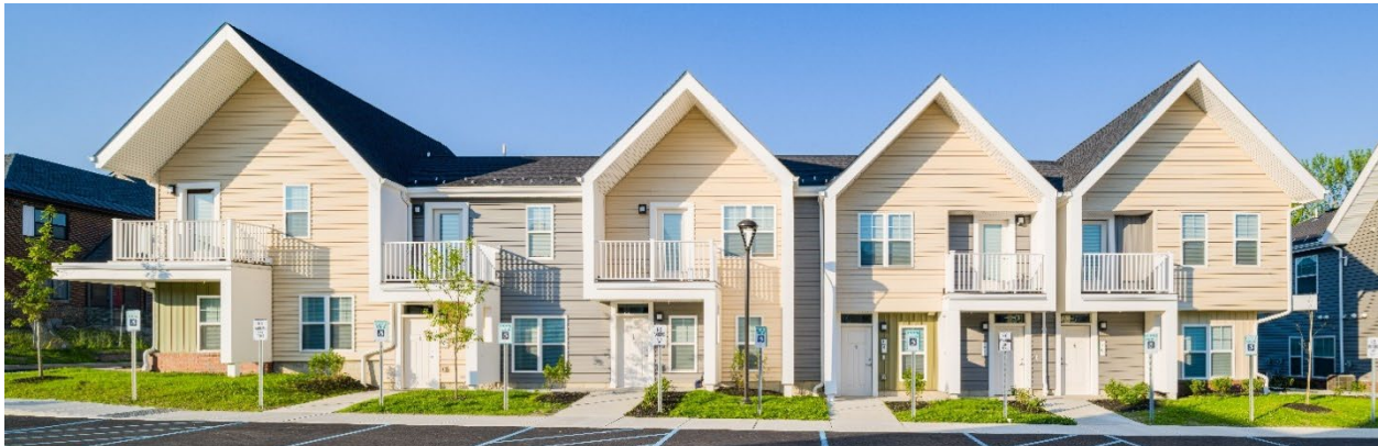
Northside Village, Schenectady, NY – Schenectady Municipal Housing Authority 300 mixed income units, 12,000 SF Community Facility Phase I completed, Phase II under construction
