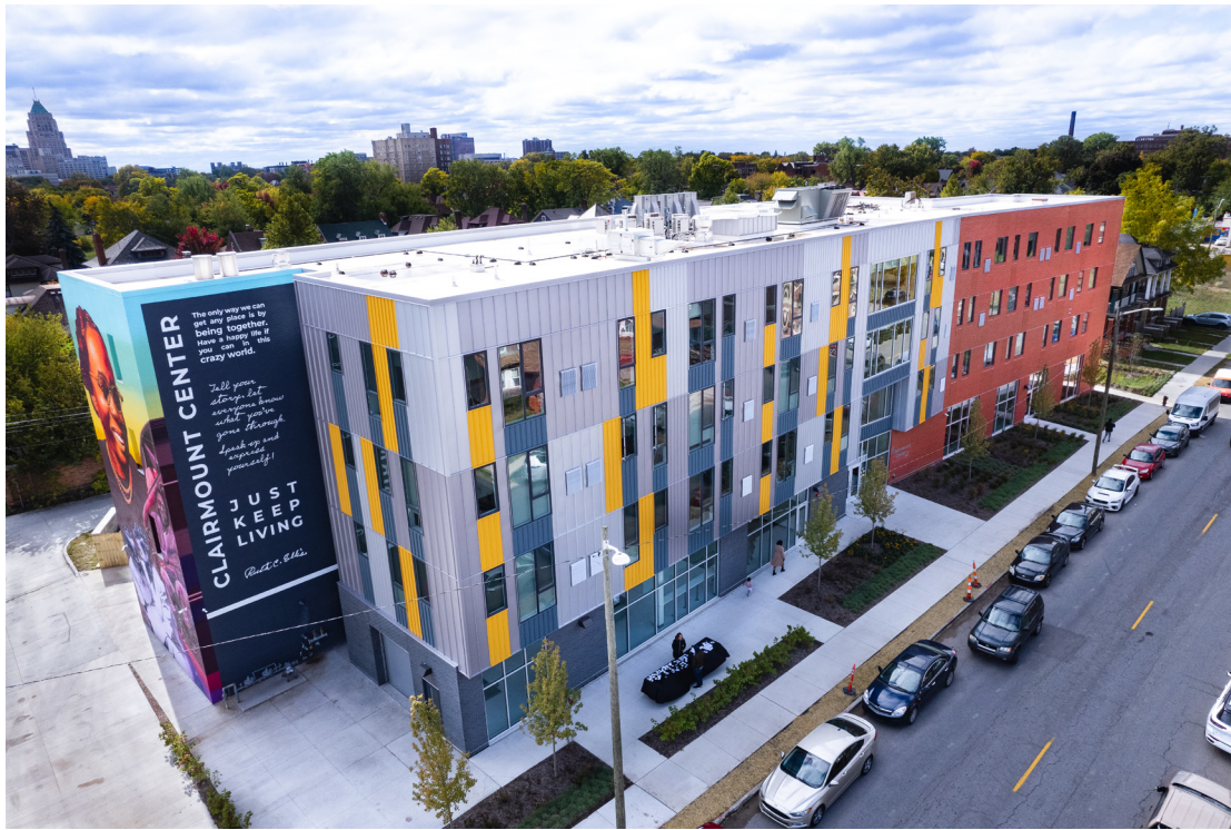
Main Facade Aerial Looking Southwest
