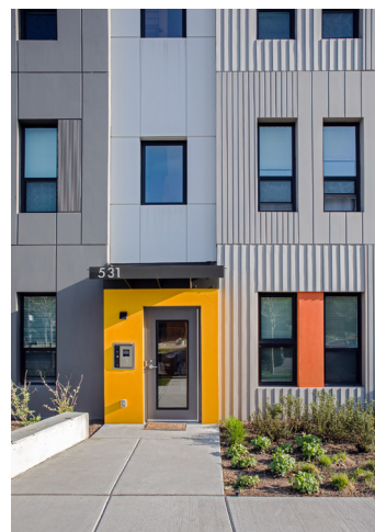
Walkup Entry Elevation
